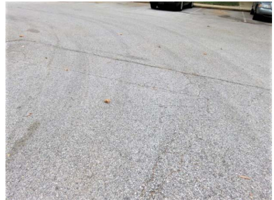
Typical asphalt pavement cracking and raveling condition
