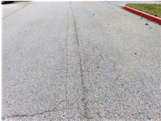
Typical asphalt pavement cracking and raveling condition
