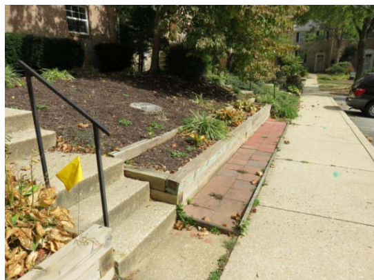
Pavers at retaining wall
