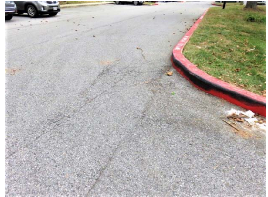
Typical asphalt pavement cracking and raveling condition
