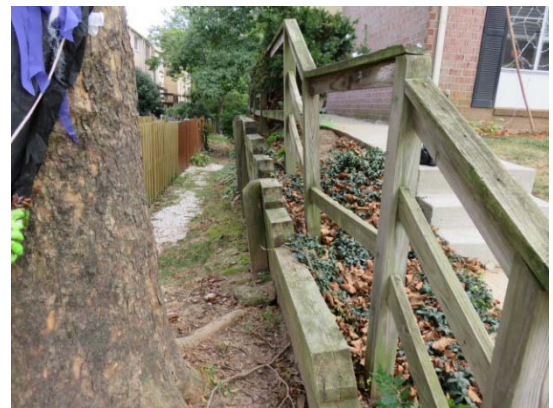
Typical wall with rot and displacement
