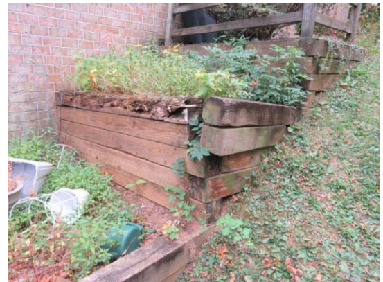
Typical wall with rot and displacement
