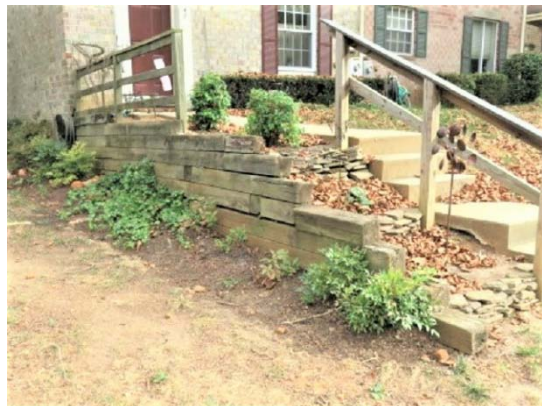
Typical loose post and missing rails
