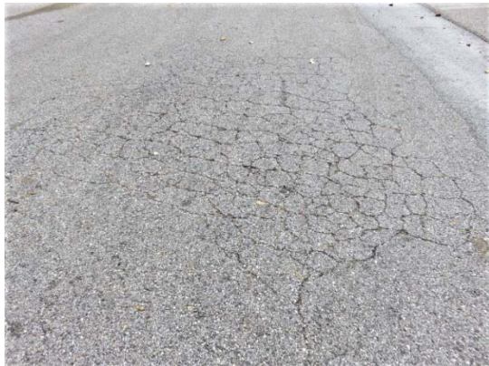
Typical alligator cracking conditions
